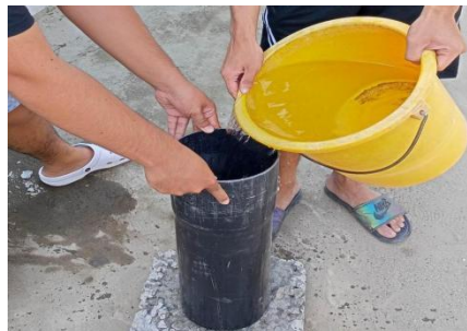
Figure 2.4.2 Pouring of water to the concrete
