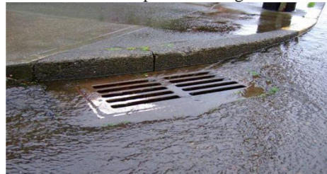
Figure 2.5.2.1 Road surface drainage
