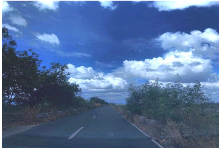
Figure 1.2: Street View of Sta. Rita and Porac Mega dike in Pampanga
