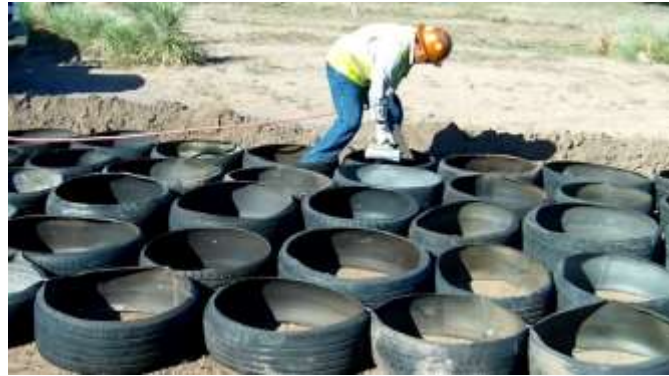
Figure 3: Jointing Tires Together By Using Heavy Duty Stapler
