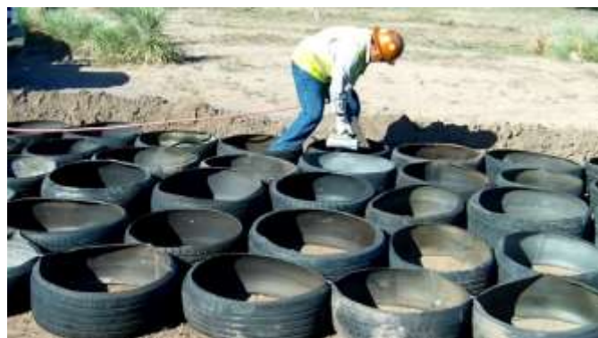
Figure 6: Jointing tires with the staple
