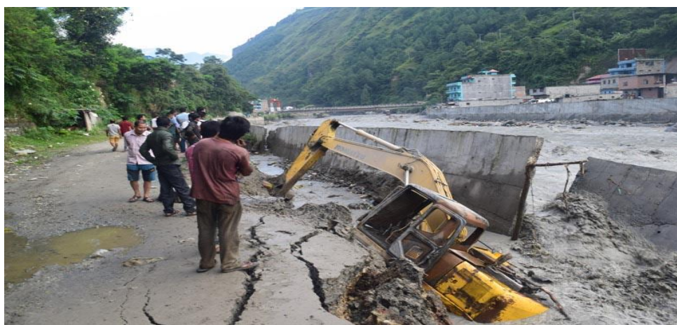
Figure 2: A road near Beni Bazaar at risk due to erosion caused by the flood in Kaligandaki River, in Myagdi, on Thursday, September 13, 2018. (Photo: THT)
