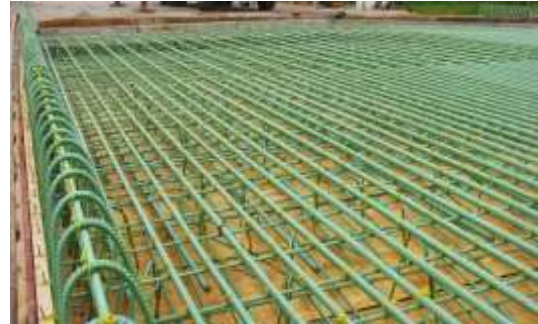
Figure 2: Epoxy Coated Reinforcing
