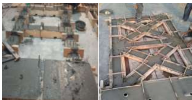
Figure-1: Casting of RC Frames
