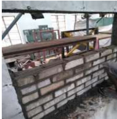
Figure-2: Construction of Reinforced Aerocon Block Infill
