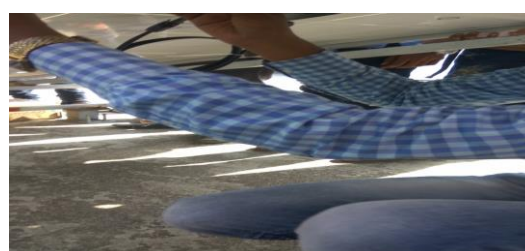
Fig. 2 Installing the panels and wiring
