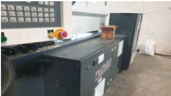
Machines were found coated with dust and oil stains which were not cleaned by the operator or any cleaning staff
