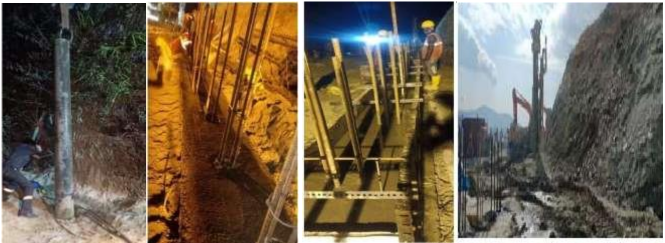
Fig. 2: Installation of Zinc-Chromium coated stainless steel cased micropiles at Mangan site.
