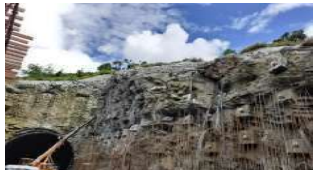
Fig. 10: Installed post-tensioned cable anchors near tunnel passage
