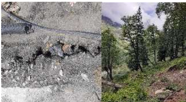
Fig. 3: Site observation made at critical location
