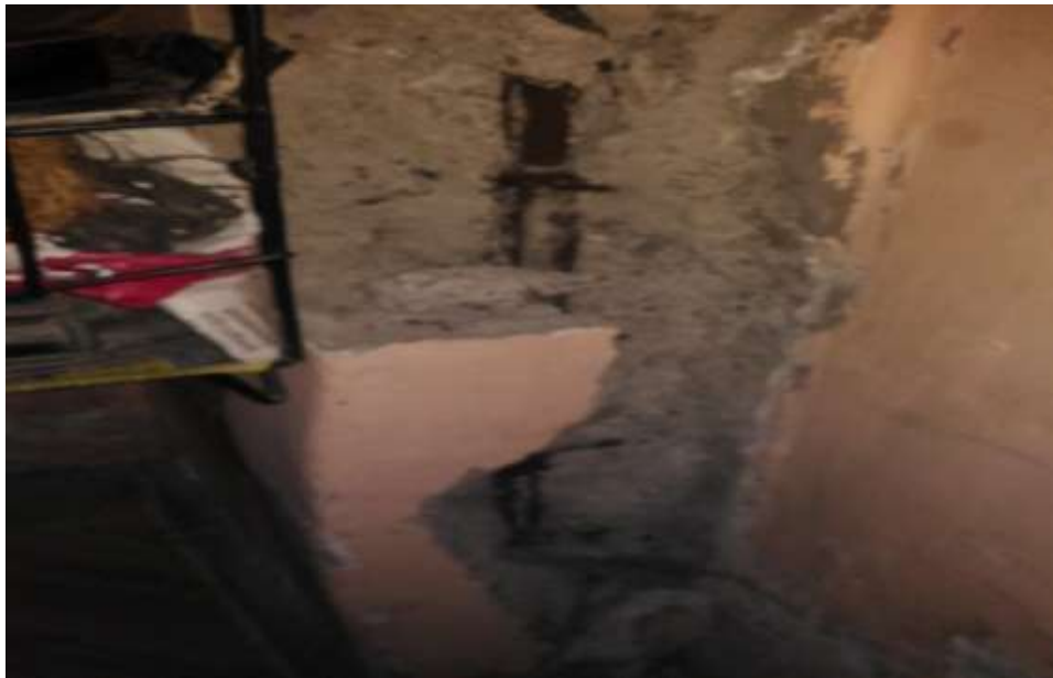
Exposed reinforcement.
