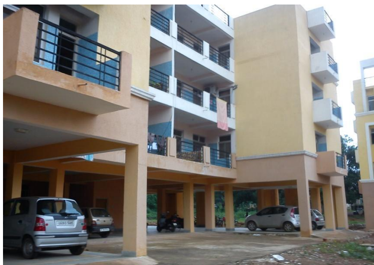
Fig. 1: Typical Open Ground Storey Building
