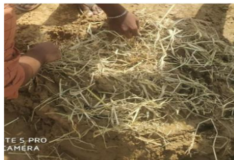
Fig. 3: Addition of strawbale
