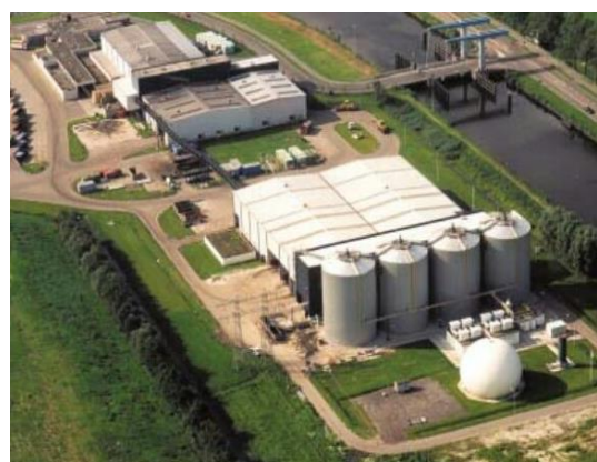
Fig. 5: Vagron Plant (Groningen) for separation and digestion of the organic fraction of MSW
