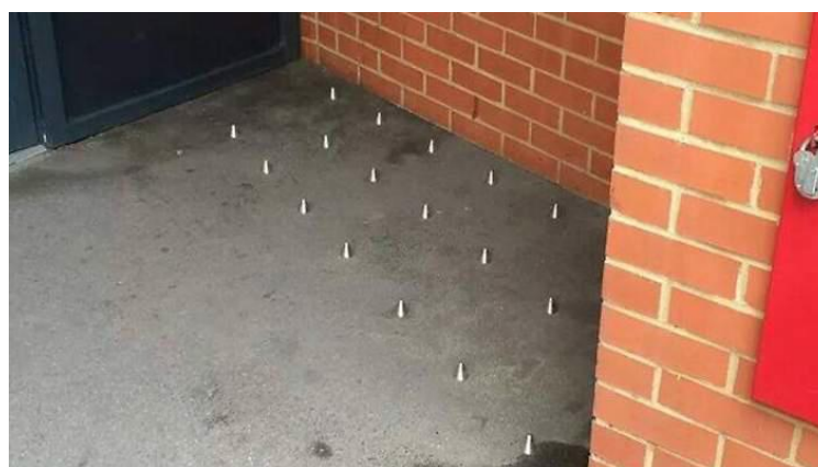
Fig. 10: Anti-homeless' spikes installed in an apartment building entrance in South London
