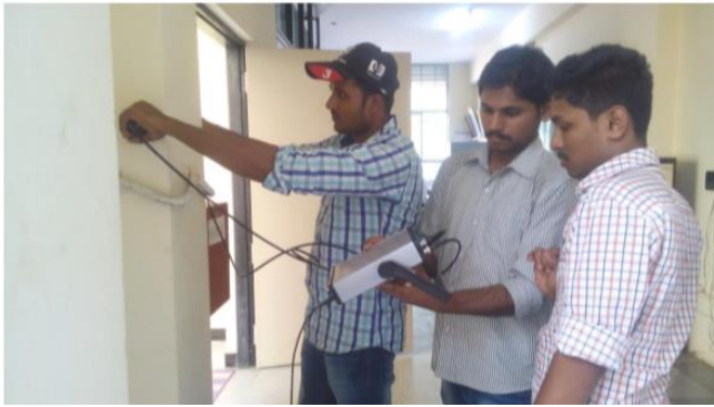
Fig. 6: Performing ultrasonic pulse velocity test on the column
