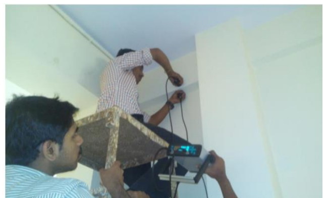
Fig. 5: Performing ultrasonic pulse velocity test on beam
