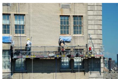
Fig. 4: Suspended Scaffolding
