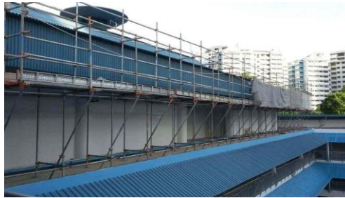
Fig. 5: Cantilever Scaffolding
