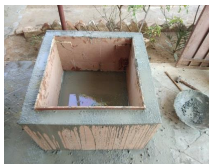
(e) Fig. 4(e) Constructed model tank
