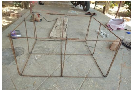
(a) Fig. 4: (a) Reinforcement work
