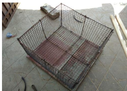
(c) Fig. 4: (c) Completed reinforcement work
