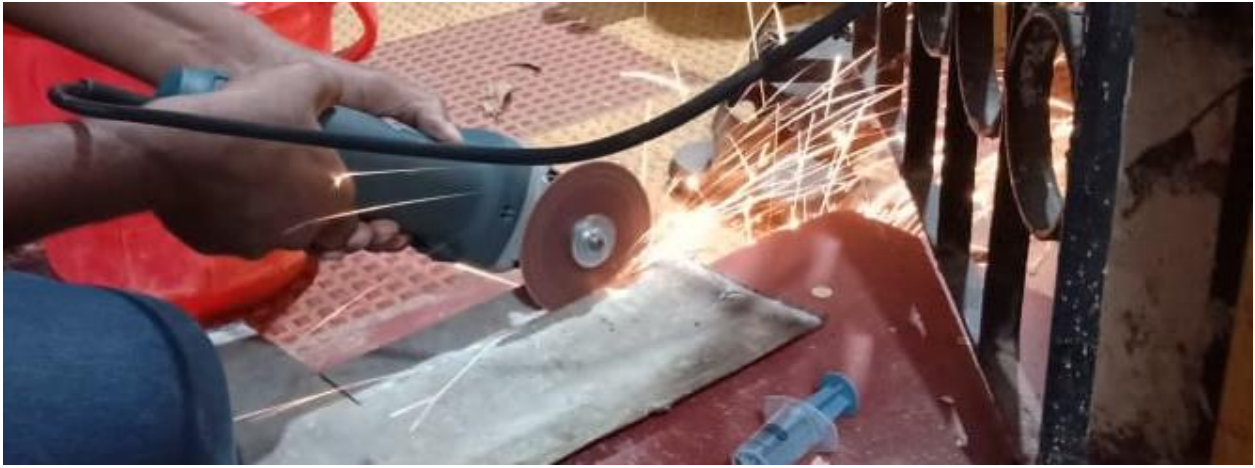
Fig. 4.1 Cutting of Mild Steel Sheet
