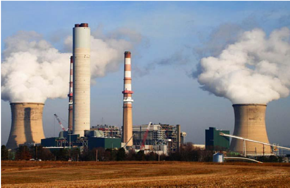
Fig. 1: Self-supporting Steel Chimney
