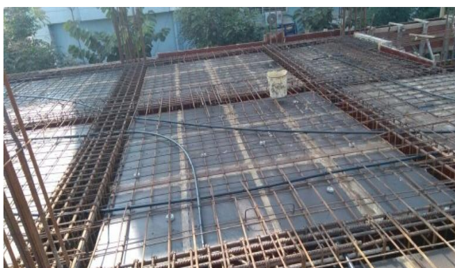
Fig. 6: Pictures of concreting on site
