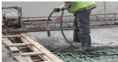
Fig. 10: Concrete compaction procedure
