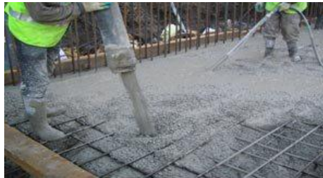
Fig. 5: Concrete laying procedure
