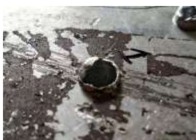
Fig. 20: Drilling at dry condition without backup support
