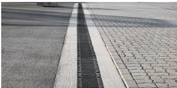
Fig. 6: Poly Propylene fiber reinforced concrete
