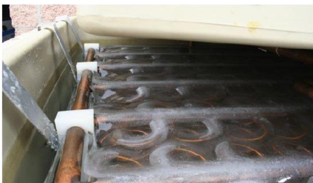
Fig. 5: Ice energy using in HVAC
