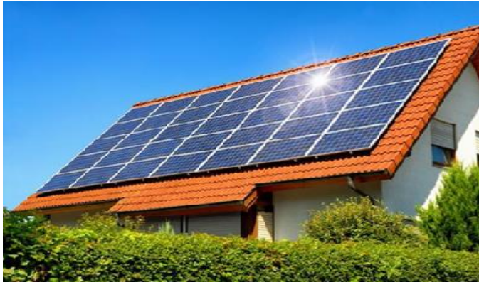
Fig. 7: Using solar power for HVAC
