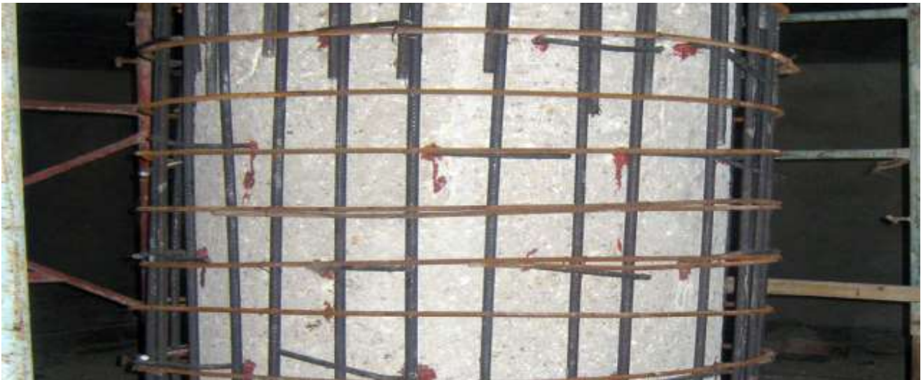
Fig. 3: RC Jacketing of Column
