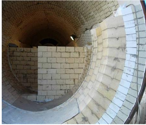
Fig.2 Refractory Inside Boiler Furnace
