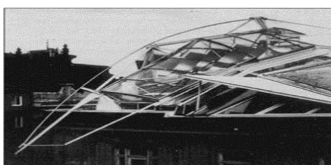
Fig.2.1: Rooftop Remodeling in Vienna, Austria, 1988
