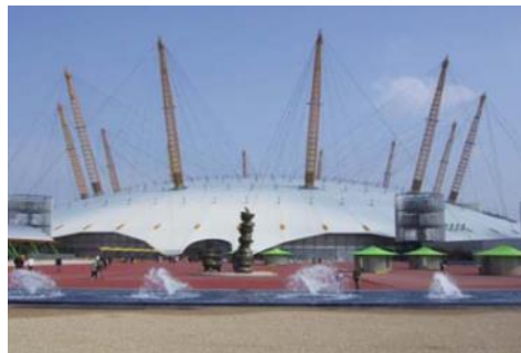
Fig2.3: The Millennium Dome
