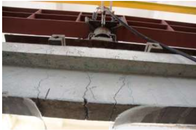
Fig: Debonding is around 21 cm and cracks occurred near the centre and under the loads
