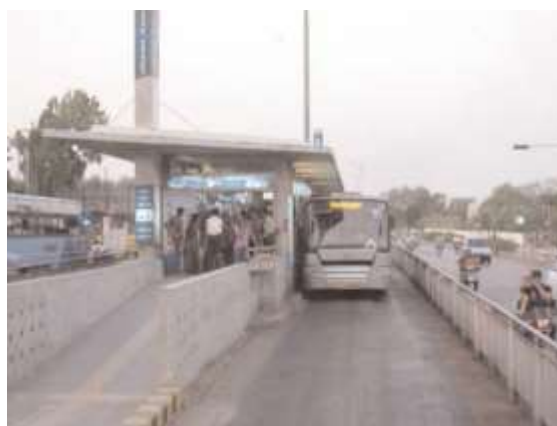
Fig 1: Janmarg BRT station in Ahmedabad.
