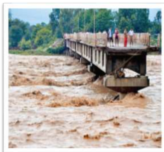
Figure: 3 Bridge Near Sangam
