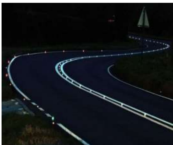
Figure 6: Solar Roadways at Night Time on the Curved Road.
