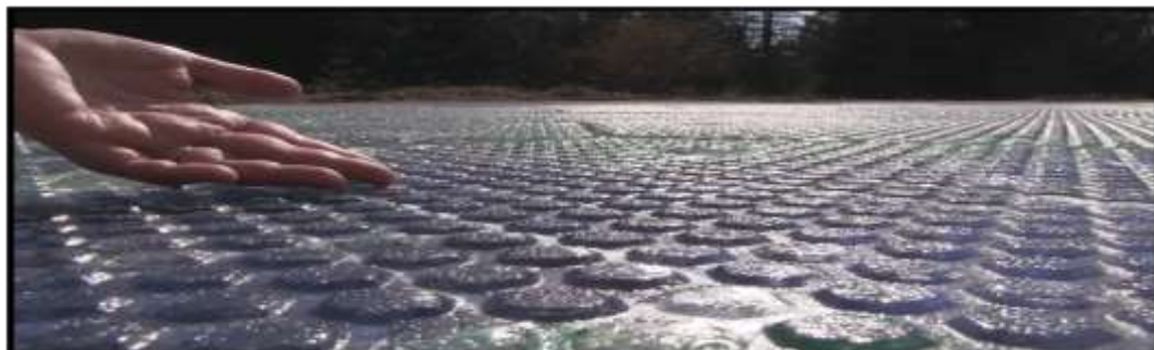
Figure 3: Road Surface Layer
