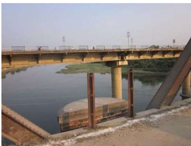
Truss bridge and simple bridge at Gomati River.
