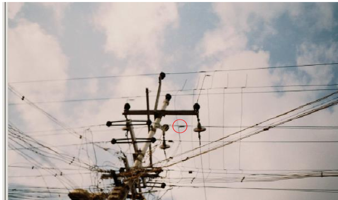
Location: Incoming to Ganthi Pottal ss Problem: improper binding location:
