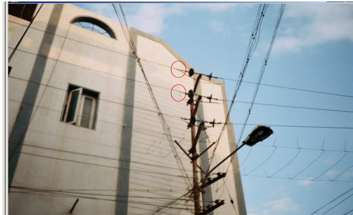
Location: incoming pole 3(Anthony moopanan ss) Problem: Imper binding& loose connection
