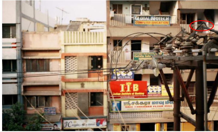
Location: DP switch Problem: flex wire damage
