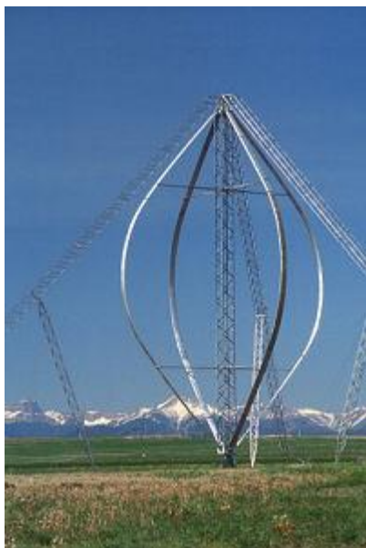
Vertical Axis wind turbines
