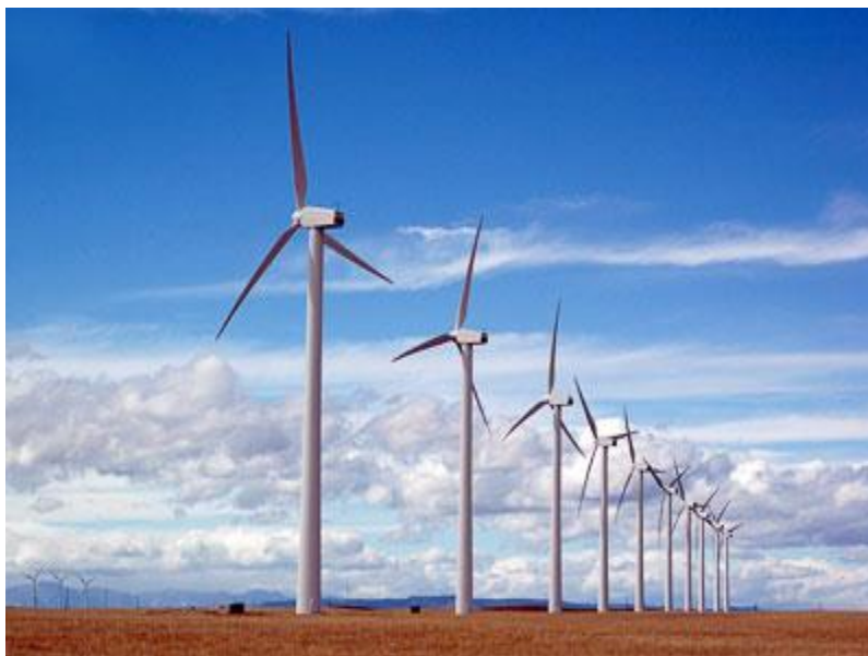
Horizontal axis wind turbines wind farm Turbines consists of three major parts
