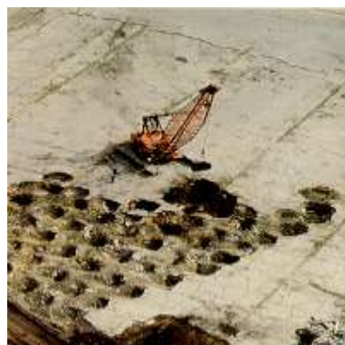
Fig: Dynamic Compaction
