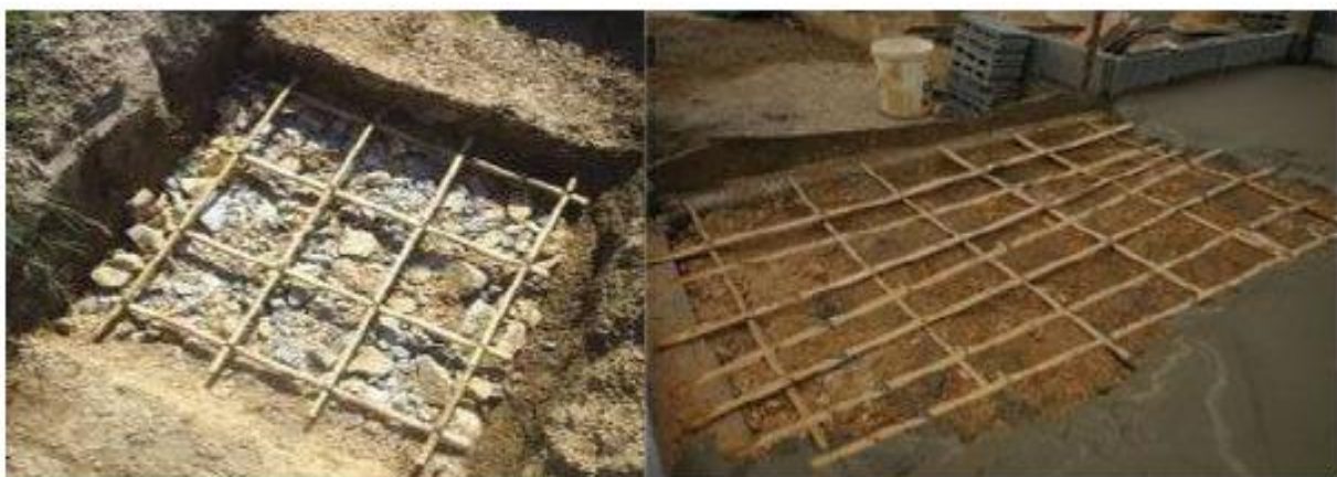
Fig. 1 Bamboo as Reinforcement
