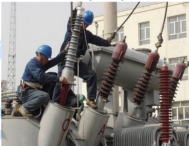
Fig.3: Bushing installation of power transformer
