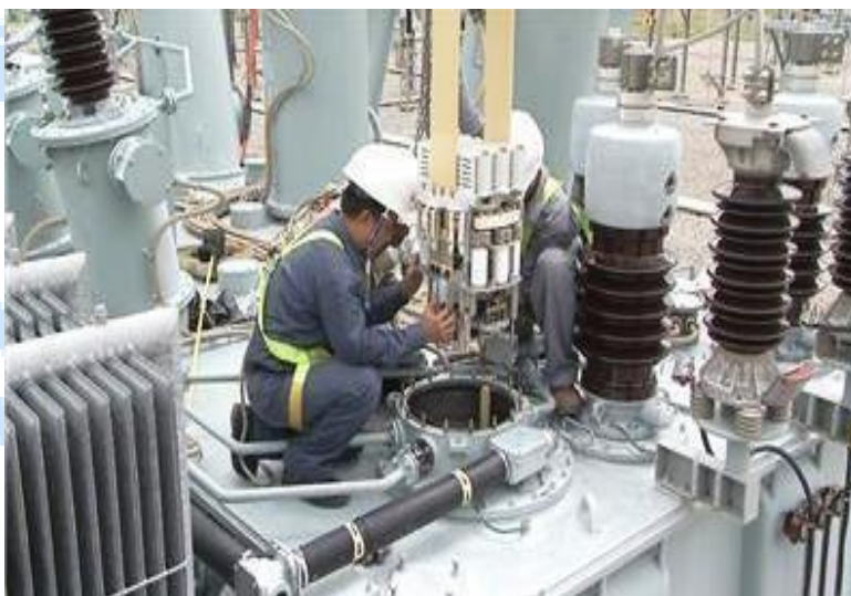
Fig.5: Tap changer Overhaul of Power transformer
