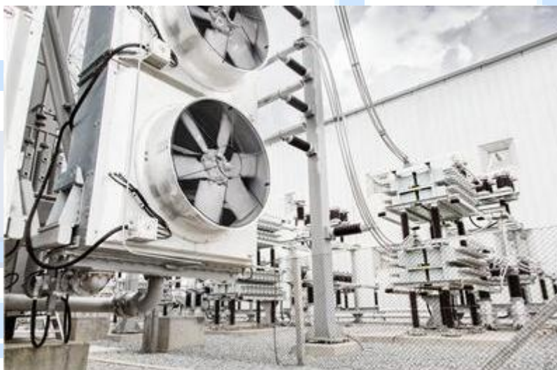
Fig.2: Example of cooling system of power transformer
